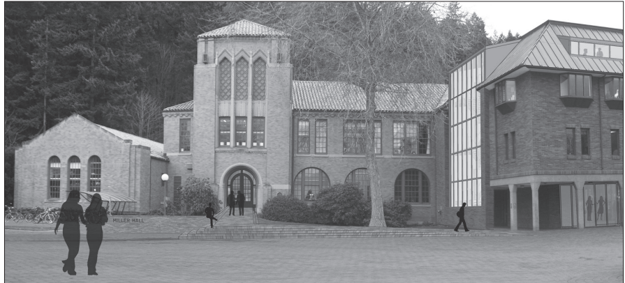
Miller Hall will get a much needed renovation with state support in the 2009-2011 Capital Budget. Miller Hall houses Woodring College of Education.
