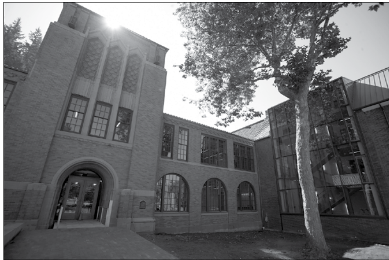
An extensive renovation of Miller Hall overhauled the entire building and added a “green roof” atop a new, glass-walled Student Collaboration Space. Miller Hall houses Woodring College of Education and the Department of Modern and Classical Languages.
