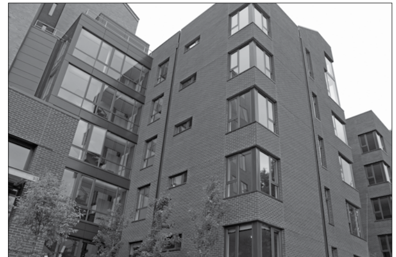
A 37,000 square-foot addition to Buchanan Towers residence hall includes room for about 100 students in suites with living areas, study spaces and kitchenettes. The project is designed to achieve a LEED Silver rating.
