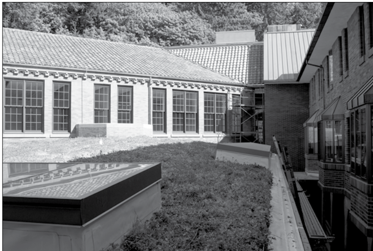
A new green roof tops Miller Hall's new Student Collaboration Space.
